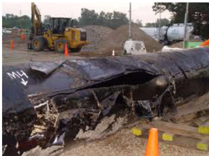
The 2010 pipeline spill in Marshall, Michigan (Kalamazoo) has cost almost $1 billion to clean up and is still not finished.
